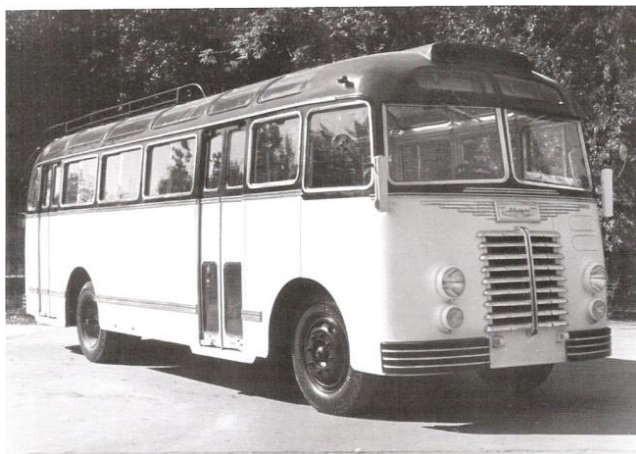
Ikarus 30: the first self-supporting bodywork vehicle
